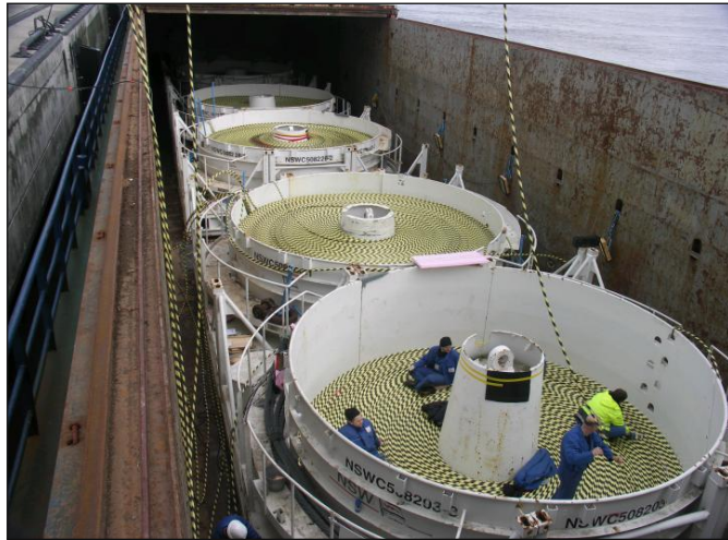
Winding of the cable in the cable container
