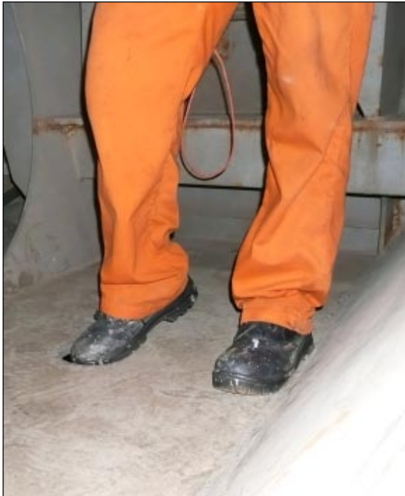
Holes in the platform where a shoe may be tripped
