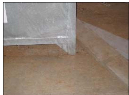
The metal “feet” of the bins
