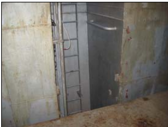
How to enter the tween deck from the ladder
