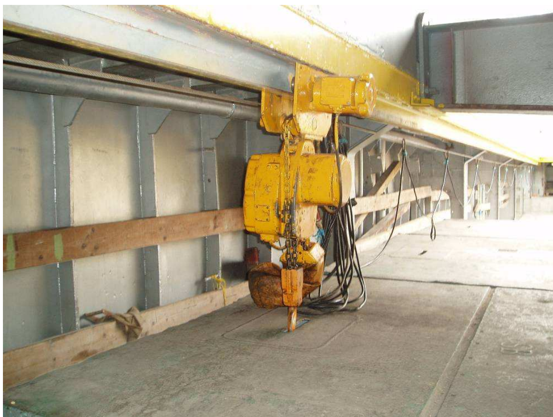
KITO crane (pulley) for removal/shifting pontoons
