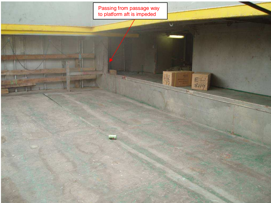
Tween-deck seen from port side, pontoon number 19 is closed
