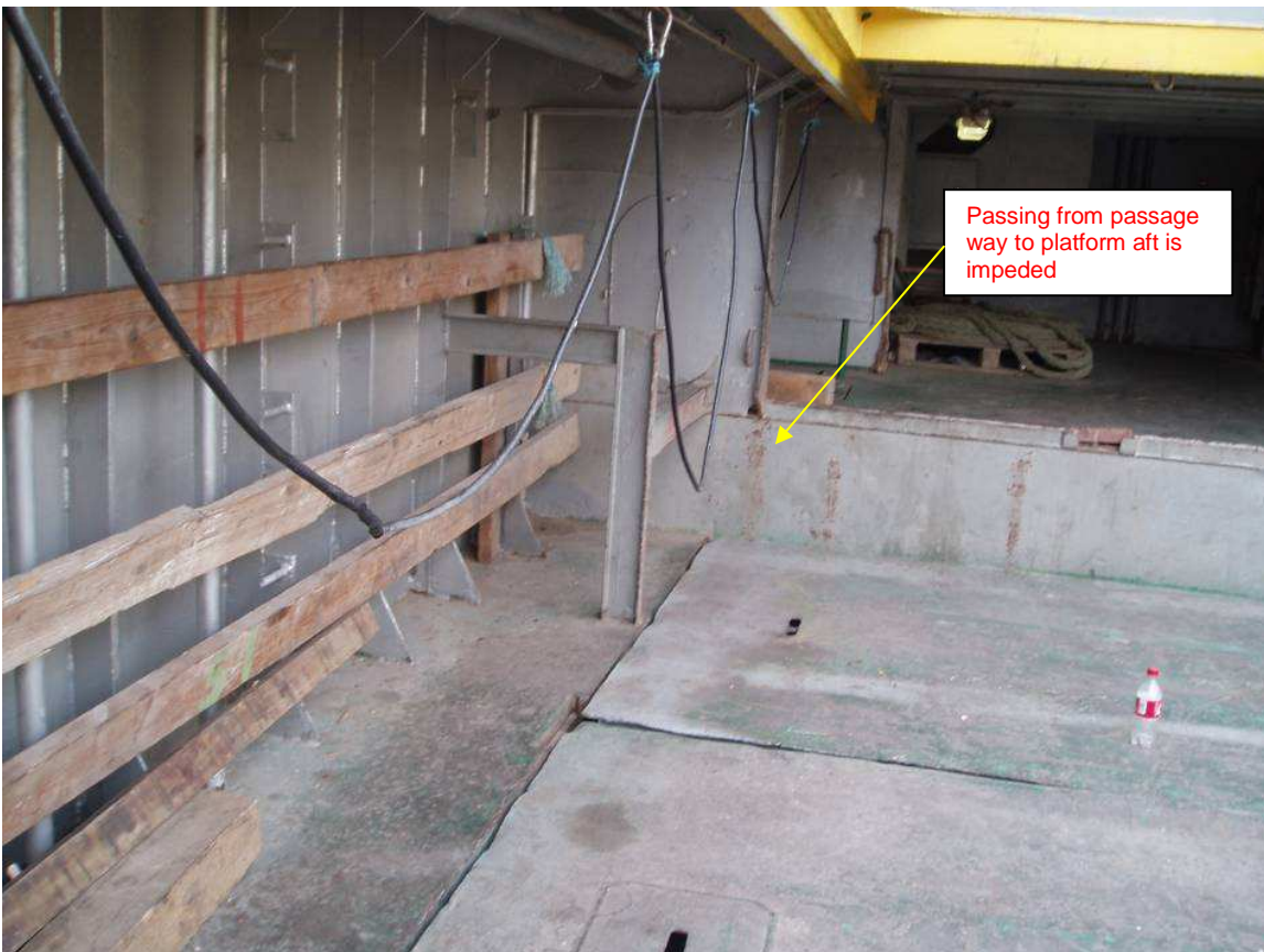
Tween-deck and passage way, starboard side.
